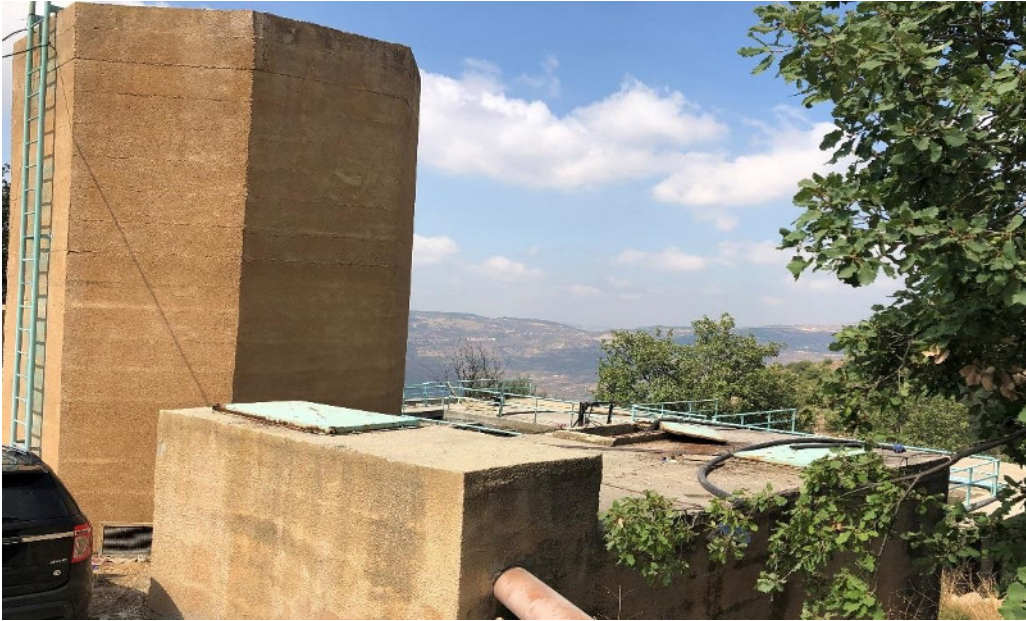
Figure 90. Jbaa wastewater treatment plant
