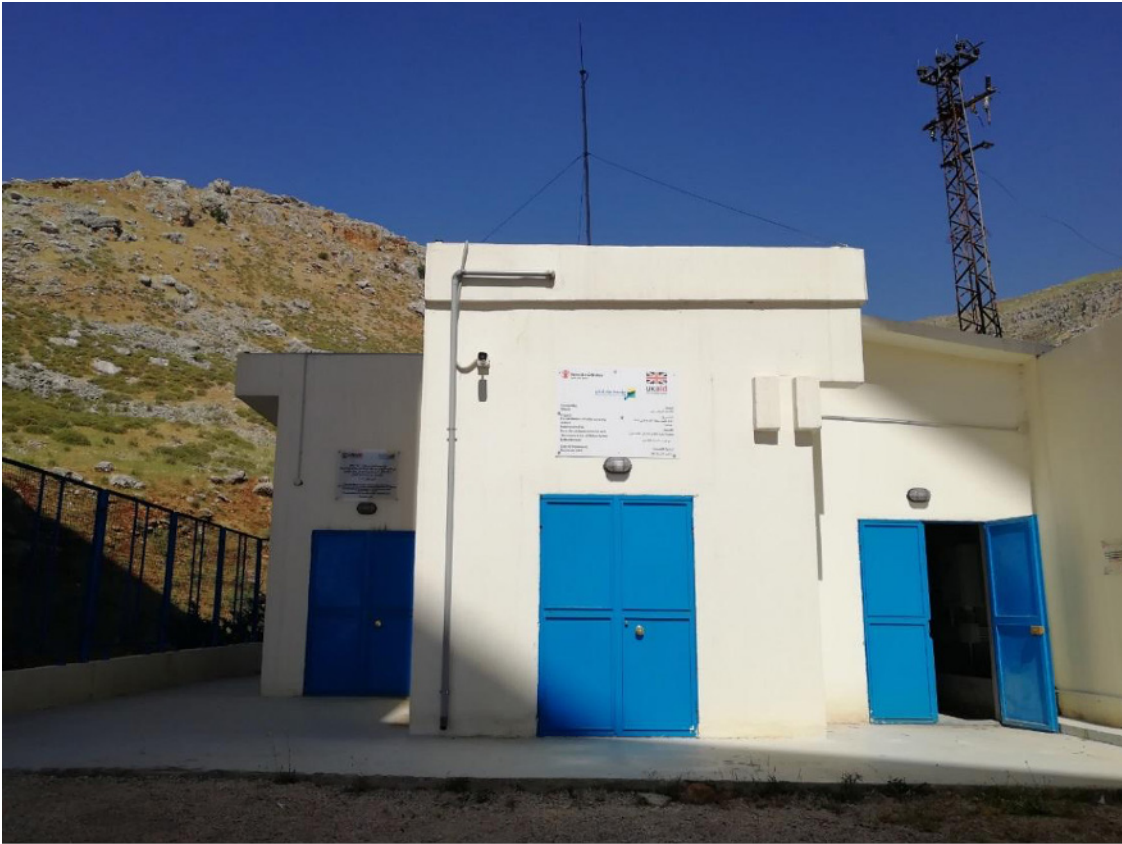
Figure 35. Jdita water pumping station
