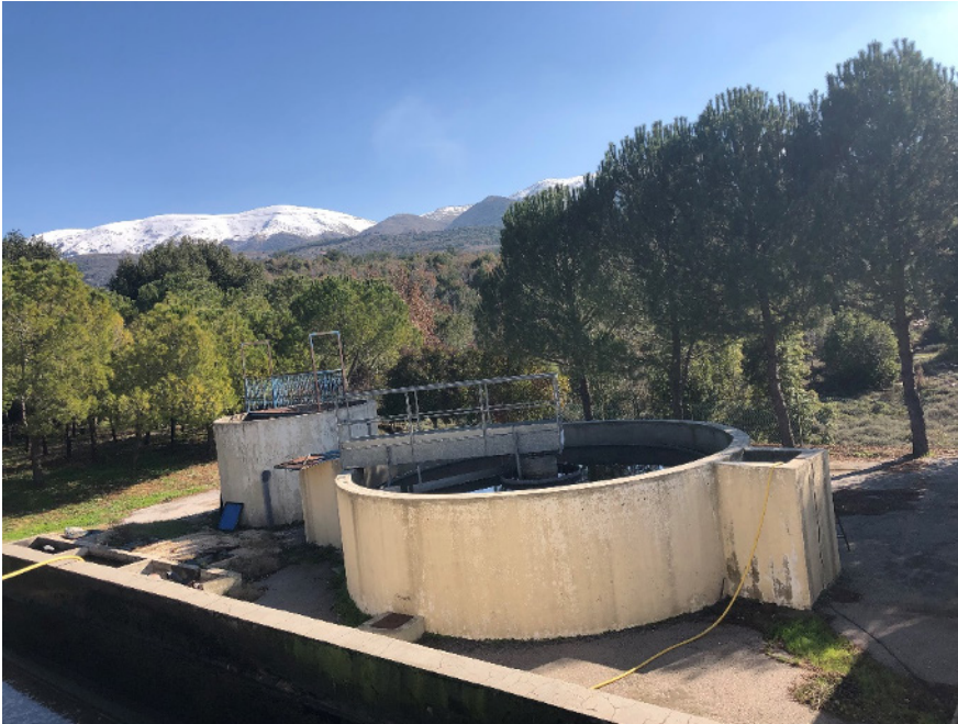
Figure 92. Baadaran wastewater treatment plant
