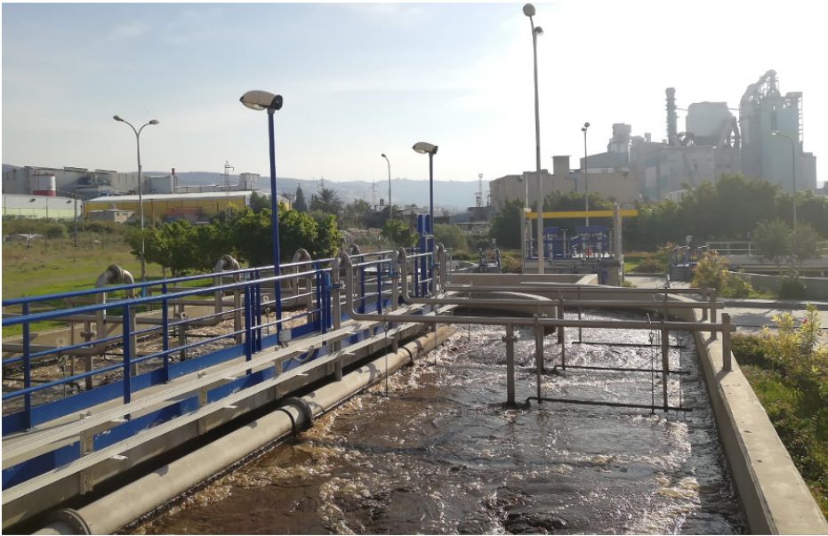
Figure 97. Chekka Wastewater Treatment Plant
