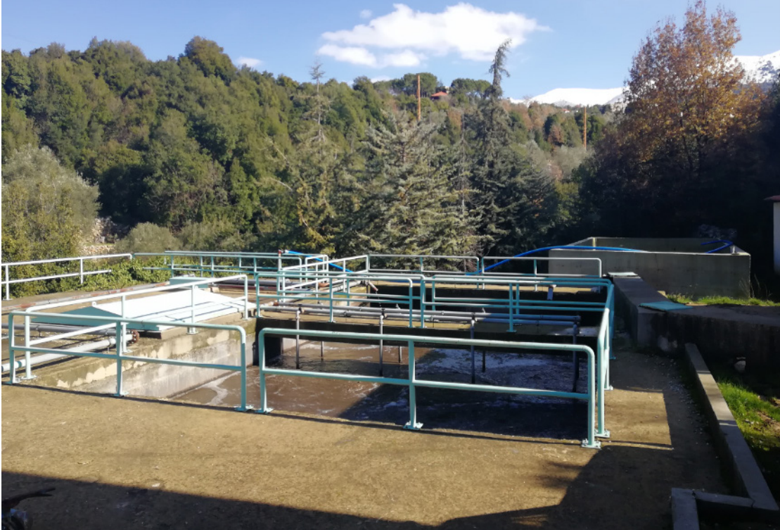
Figure 93. Khraybeh wastewater treatment plant
