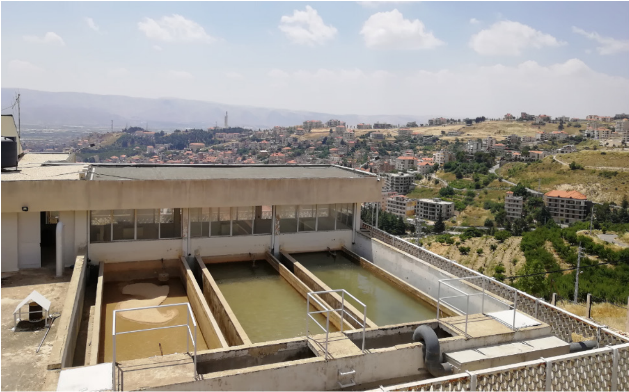
Figure 38. Zahle water treatment plant
