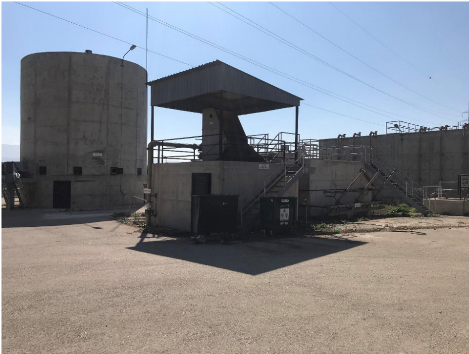
Figure 85. Ferzol wastewater treatment plant
