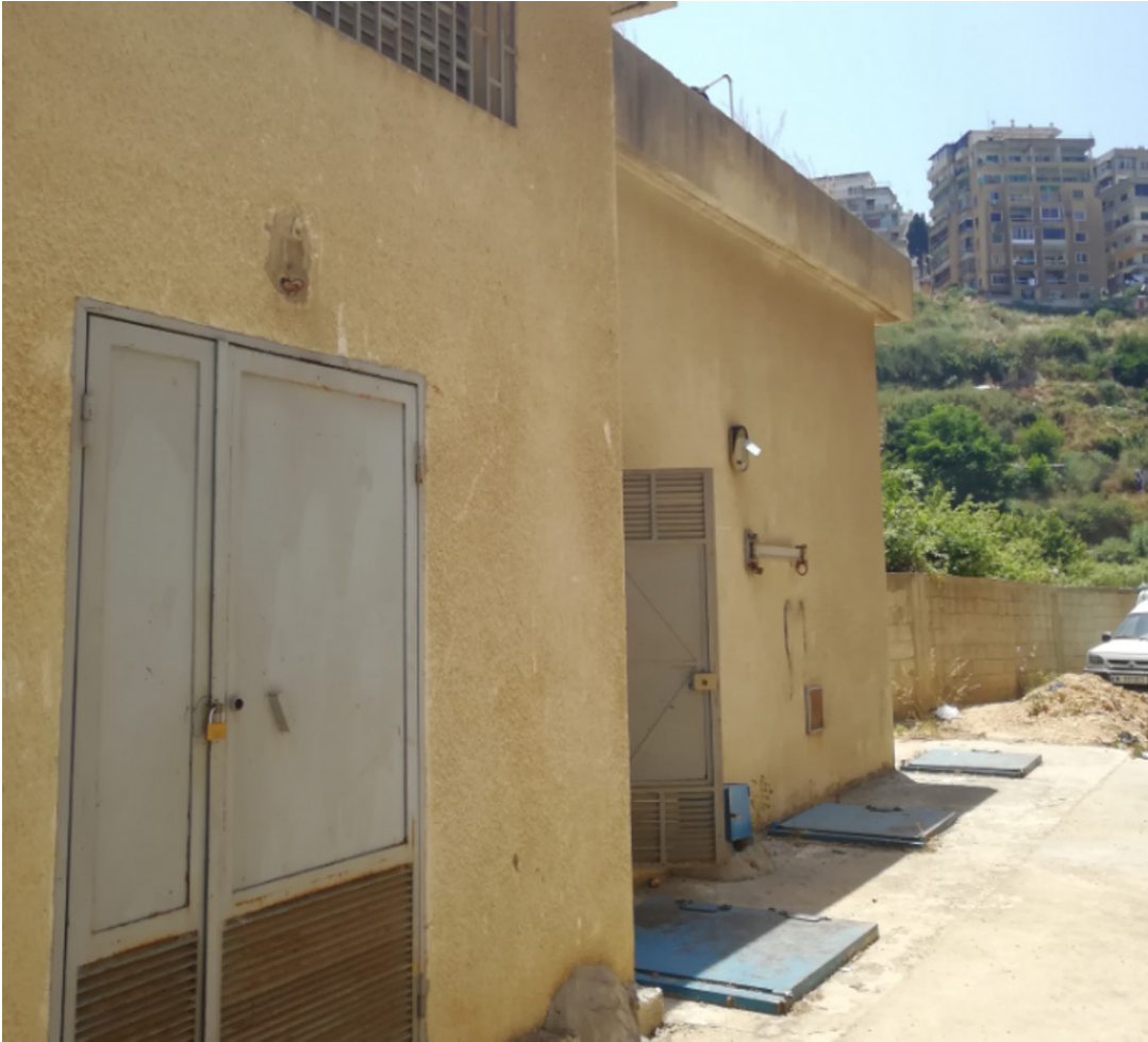
Figure 53. Jisr water pumping station
