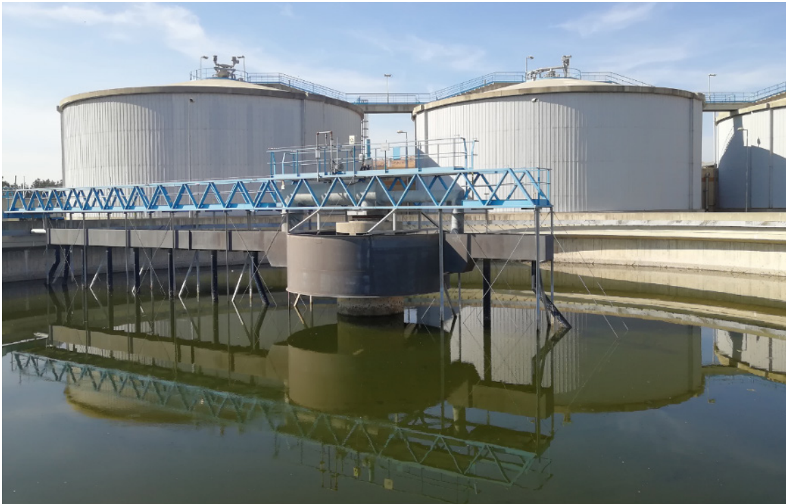
Figure 96. Tripoli wastewater treatment plant
