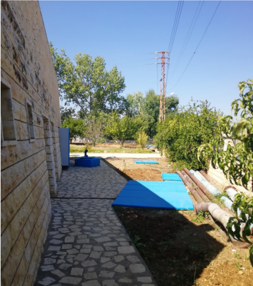
Figure 64. Al Oyoun water pumping station
