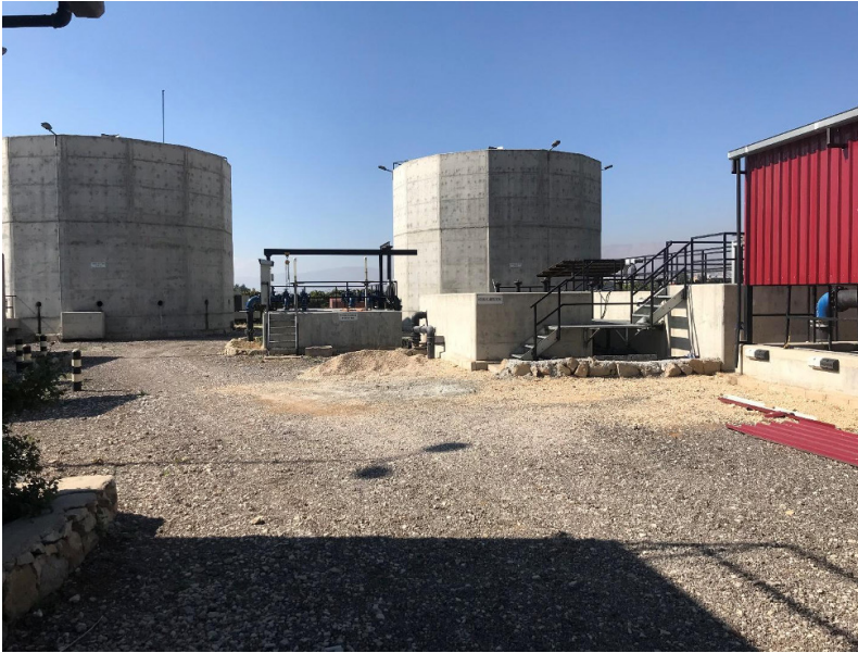
Figure 84. Ablah wastewater treatment plant
