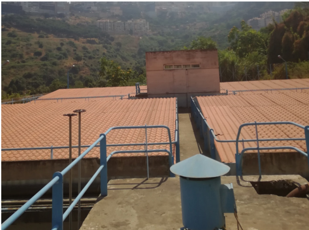
Figure 50. Dayshounieh Baabda water treatment plant
