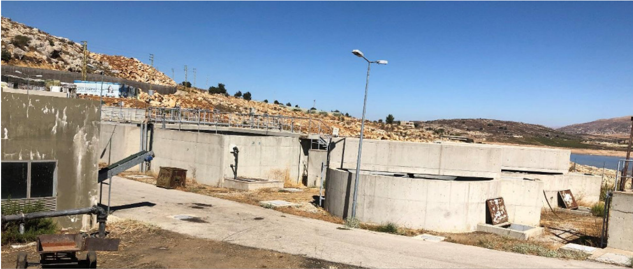
Figure 83. Saghbine wastewater treatment plant
