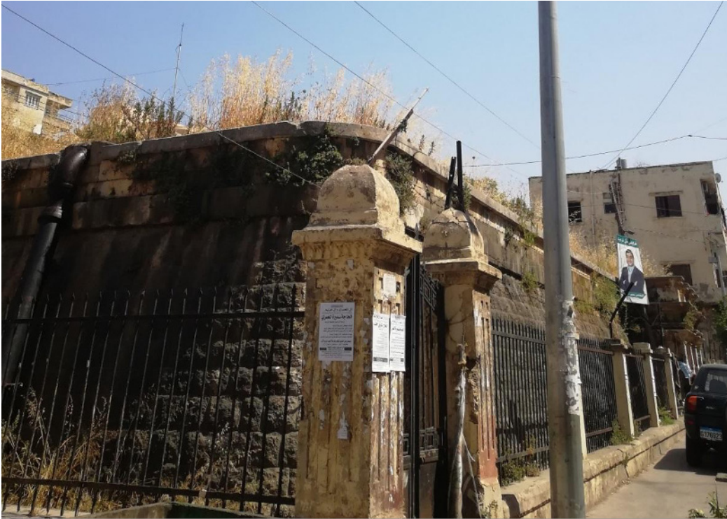
Figure 56. Daher El Moghor pumping station
