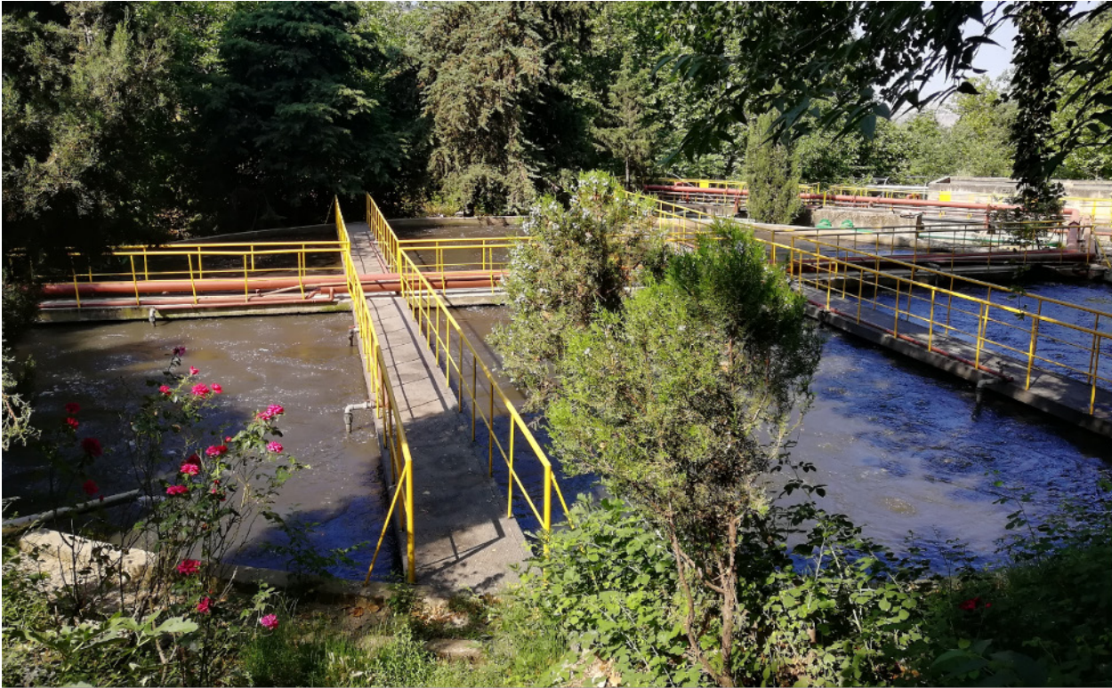
Figure 86. Hammana wastewater treatment plant
