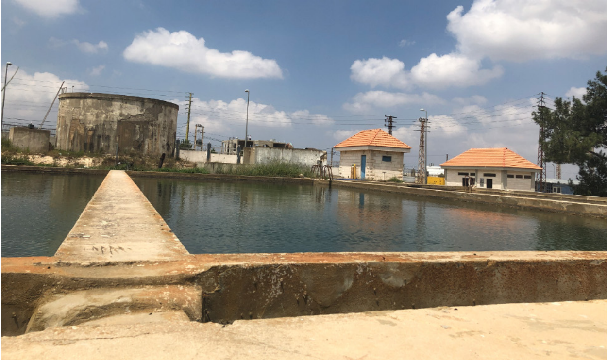
Figure 76. Taybeh water treatment station
