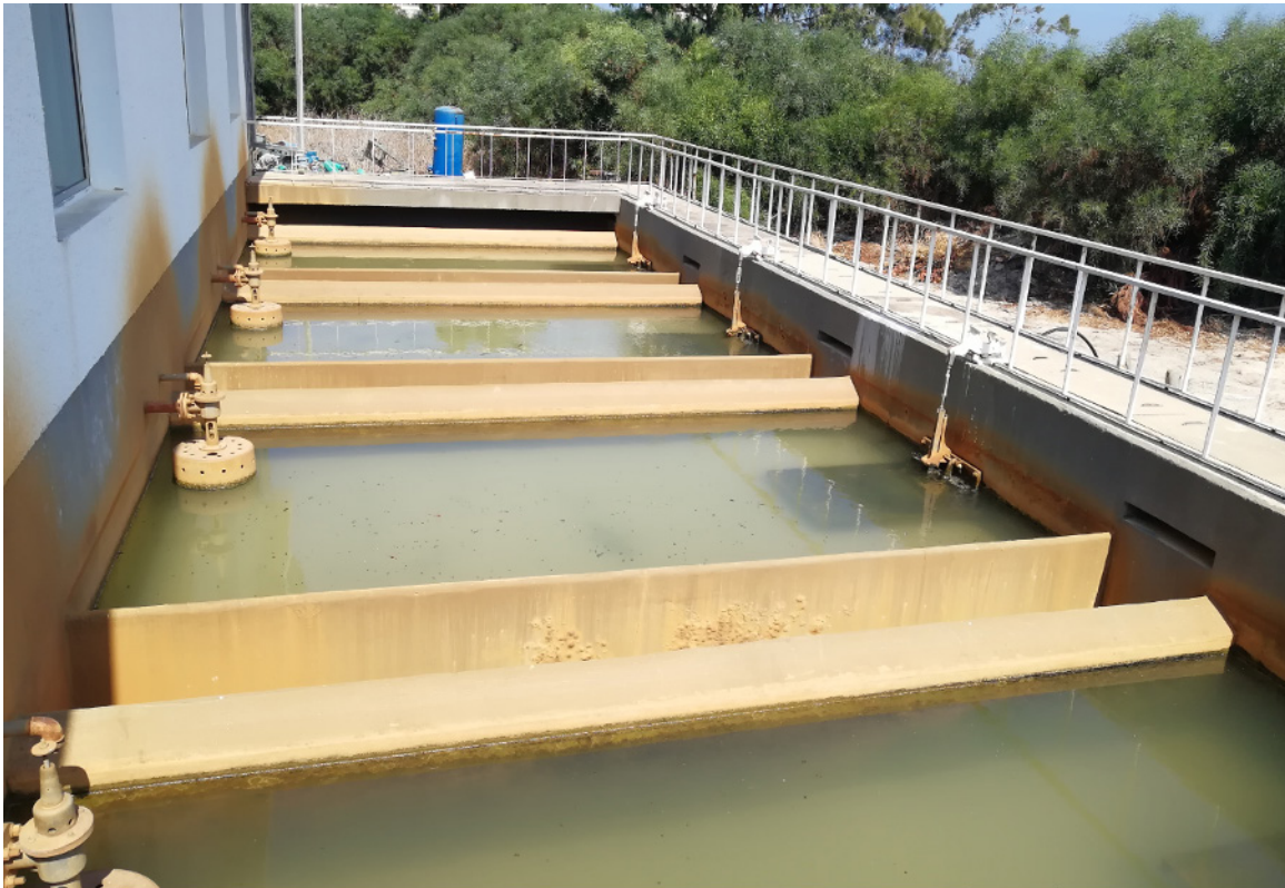
Figure 71. El Buss water pumping station
