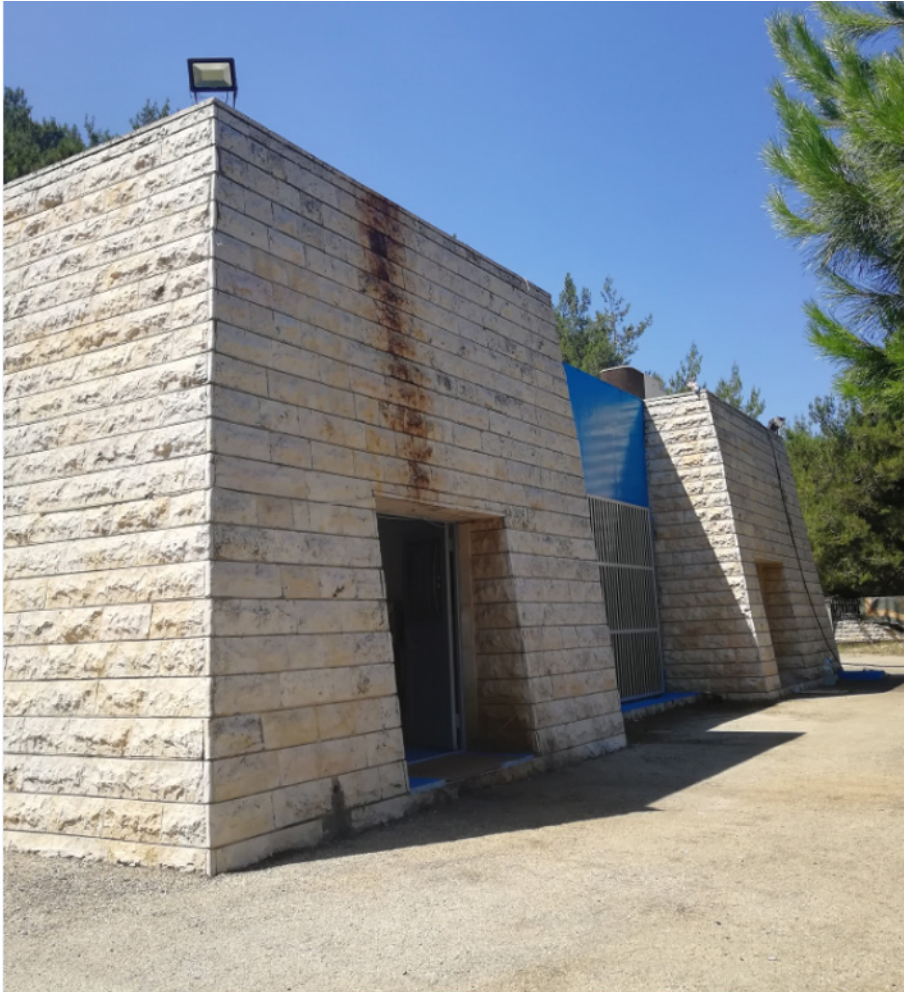
Figure 65. Ain Yaacoub Water Pumping Station
