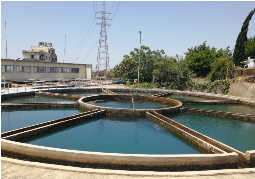
Figure 52. Bahsas water treatment plant
