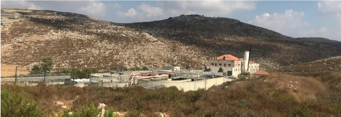
Figure 99. Nabatiyeh wastewater treatment plant
