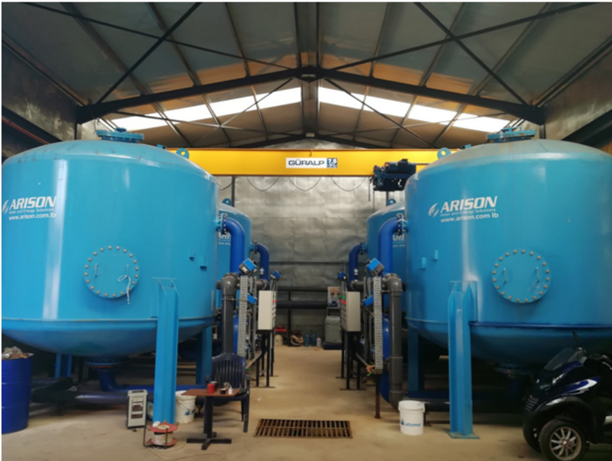
Figure 48. Reverse osmosis plant Hadath
