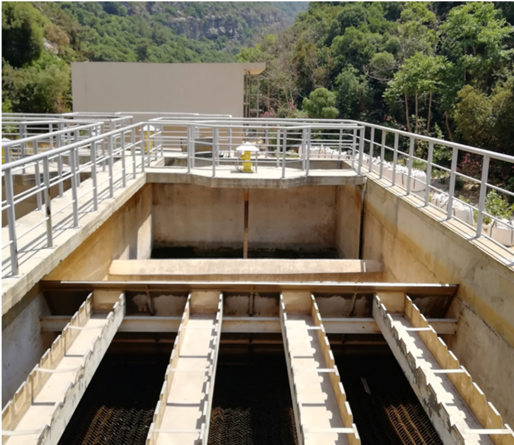
Figure 51. Dayshounieh, Metn water treatment plant
