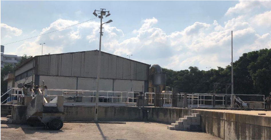
Figure 100. Sayneek wastewater treatment plant
