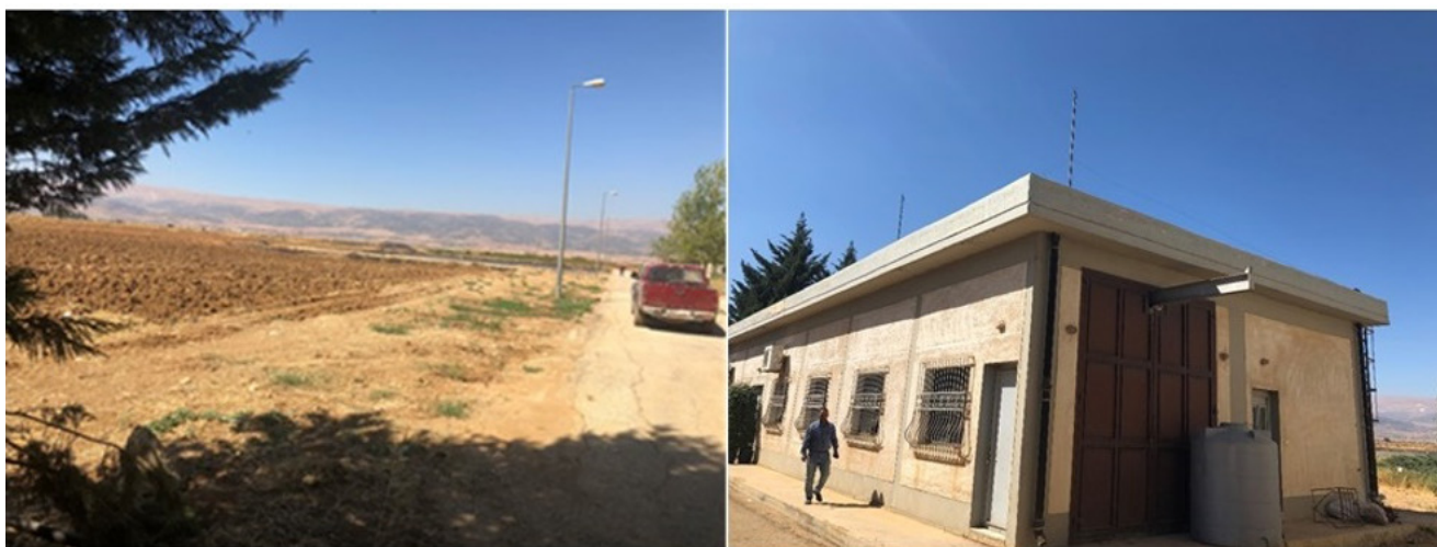
Figure 10. Available land and rooftop for solar PV installation in laot WWTP
