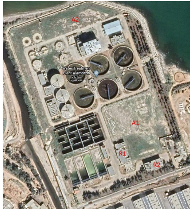
Figure 12. Available lands and rooftops for solar PV installation in Tripoli WWTP
